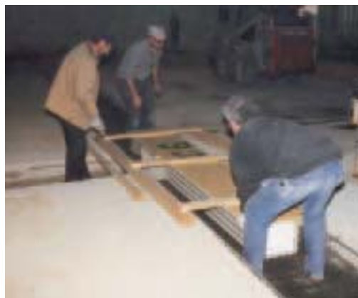
Setting of trench section
